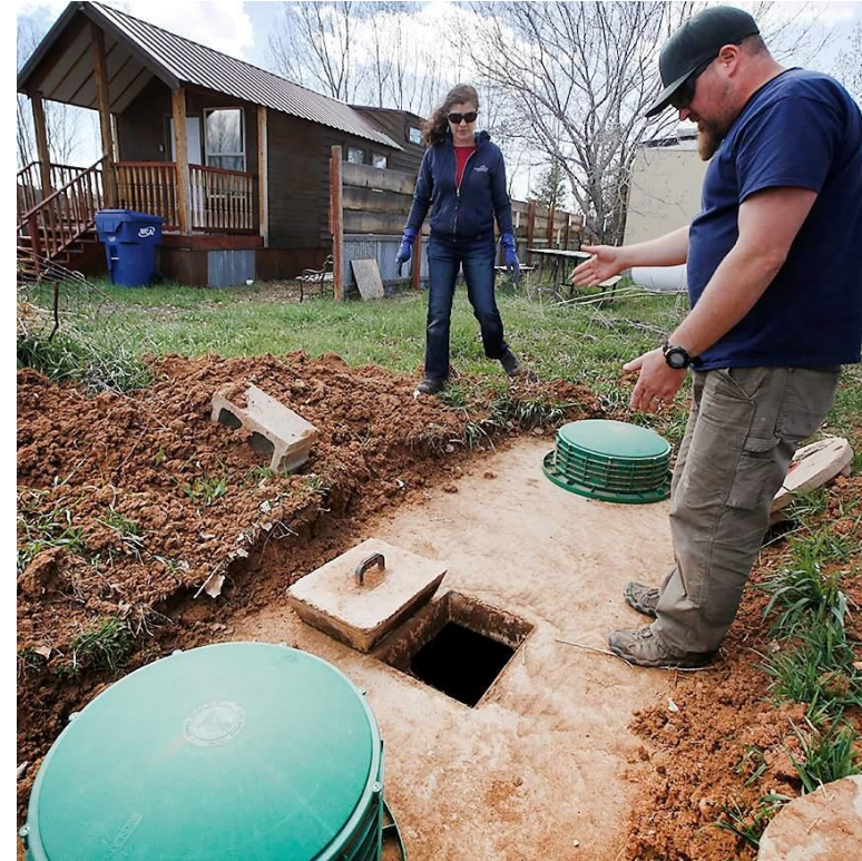
Figure 11: Septic Tank Inspection, The Durango Herald
